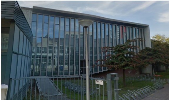
Figure 65 (left): 3mE building, lecture rooms
