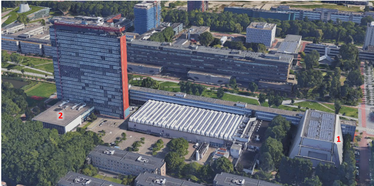
Figure 72: EEMCS building, ESP lab side roof (1) and lecture room roof (2) highlighted
