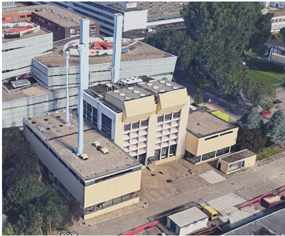
Figure 87 (left): CHP building
