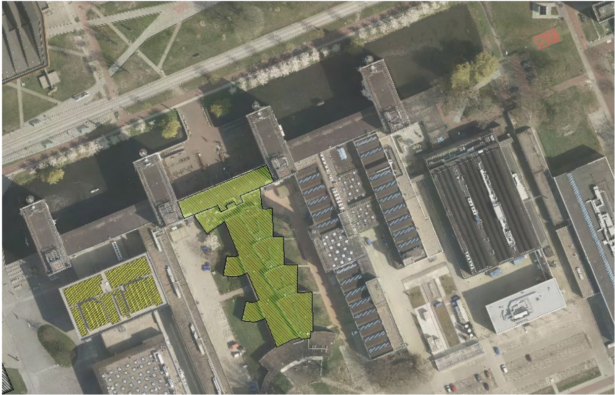
Figure 62: green roofs on the 3mE building (34)
