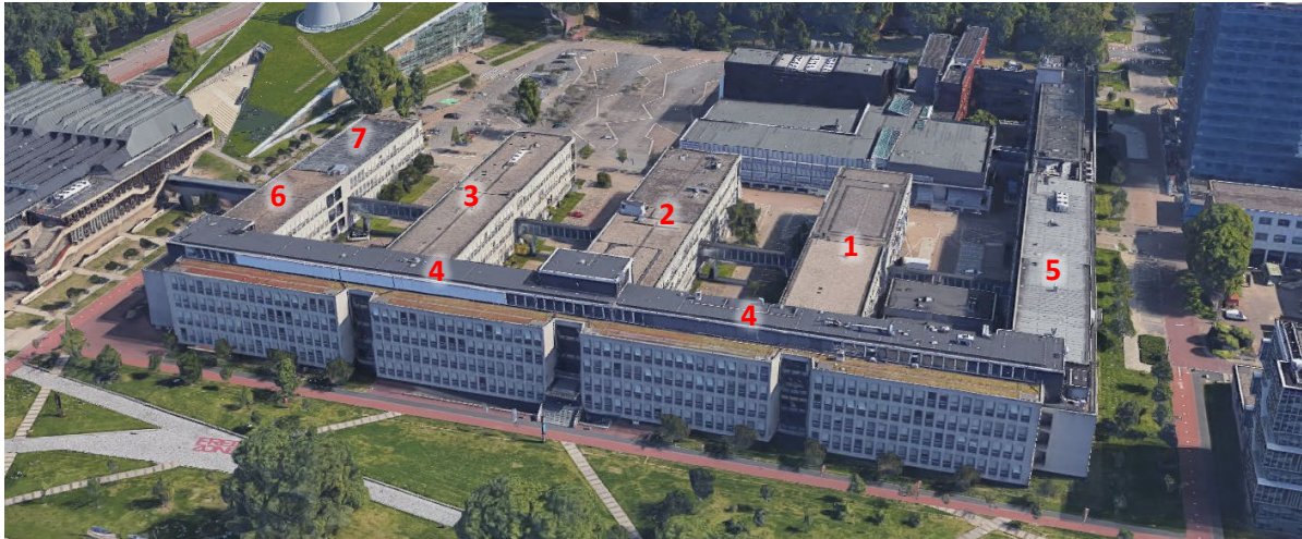
Figure 29: AS building, roofs 7 and 9 highlighted
