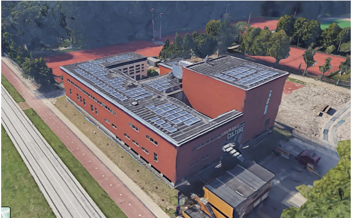
Figure 85: X Delft, building 38
