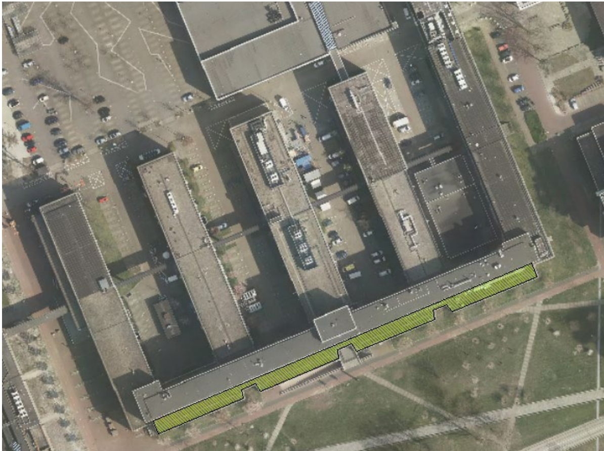
Figure 32: AS building (22), green roof
