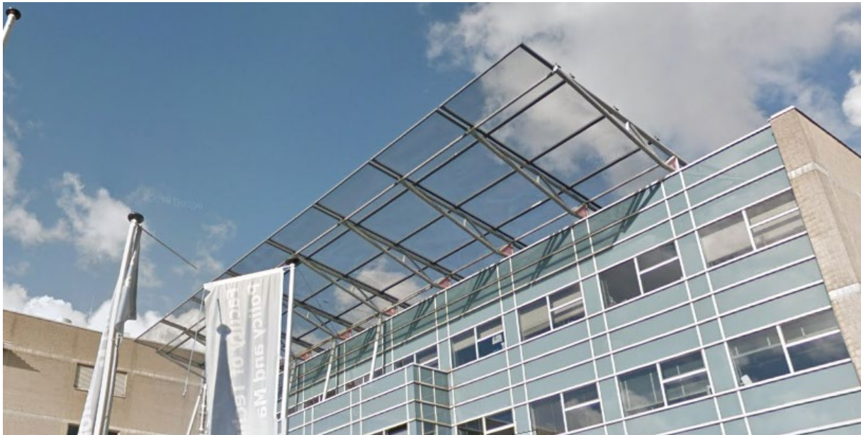
Figure 56: TPM building, canopy
