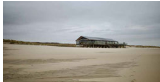
FIG. 3.29 Right: photo of the beach pavilion 'the Coast', on the left the extended deposition tail of the elevated pavilion is visible, heightening the beach and foredunes. Photo: S. Veldhuisen (2023).
