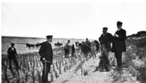
FIG. 3.44 Planting marram grass as a bio-builder for dune formation on the coast of Sylt, 1989. Source: Gerhardt, 1900.
