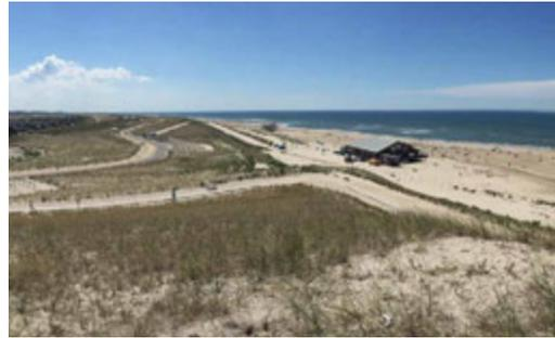
**FIG. 4.26** The coast of Petten after sandy reinforcement (2018), including a new 60 m-wide dune system.
