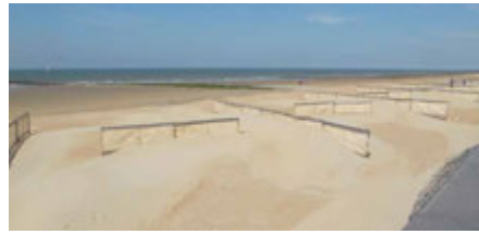
Sand screens in Belgium that could be employed for dune growth as part of the urban beach typology.
