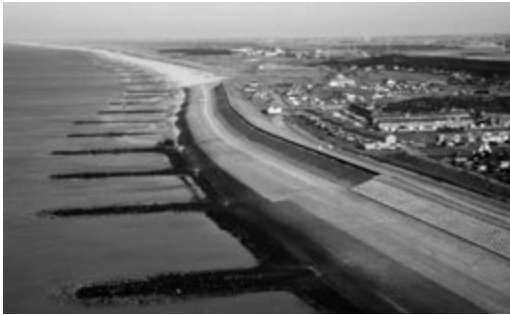
FIG. 4.25 The coast of Petten as a seawall (1980). Source: © Rijkswaterstaat.
