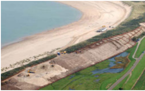
FIG. 2.9 Dune reinforcement in Renesse, NL 2014 (left). Image by the Sinke group.
