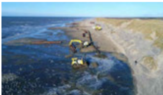
FIG. 2.6 Beach nourishment in Texel, NL 2020 (left). Source: Texelinformatie.nl.
