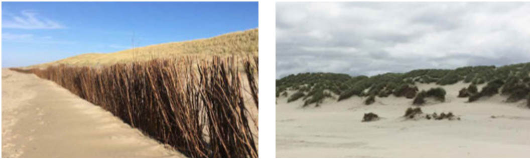
FIG. 3.41 Widening (left) or heightening (right) of the dunes requires different sediment transport mechanisms and design principles. Images by the author.
