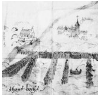
b) The village of Petten around 1552 by Jan van Scorel, with pole construction as the last sea defence.
