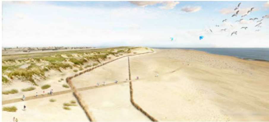
Initial fences working towards the safety buffer in the first years after reinforcement.
