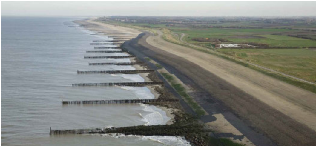
FIG. 4.23 Design study phase 0: the current seawall of Westkapelle - Domburg before BwN reinforcement. Photo: © Rijkswaterstaat / Rens Jacobs.
