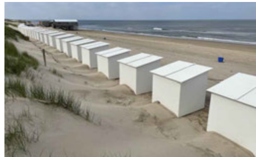
FIG. 3.31 Photograph of the beach row housing and pavilion of Camperduin after sandy reinforcement. Sediment is transported between the gaps against brushwood fences. Image by the author.
