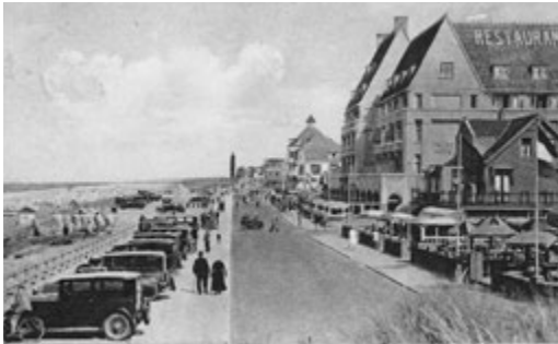
FIG. 4.2 Photograph of the Noordwijk boulevard in 1920. Source: deoudedorpskernnoordwijk.nl.
