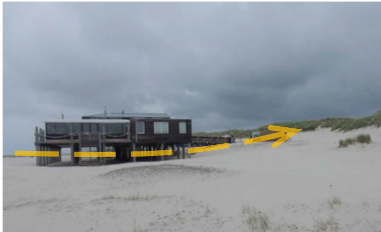
FIG. 3.78 Compressed, accelerated windflow below and behind a beach pavilion on poles to increase sediment flow to the dunes. Image by the author.
