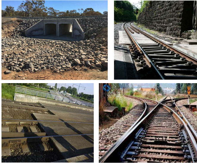
Figure 1.4: Different types of transition zones in railway tracks. Culvert (top left; source: https://joewagnergroup.com.au/projects/western-culverts-replacement/ ), tunnel (top right; source: [12]), bridge (bottom left; source: [4]), and switch (bottom right; source: http://www.railroadpart.com/rail-track-parts/railway-turnout.html ).
