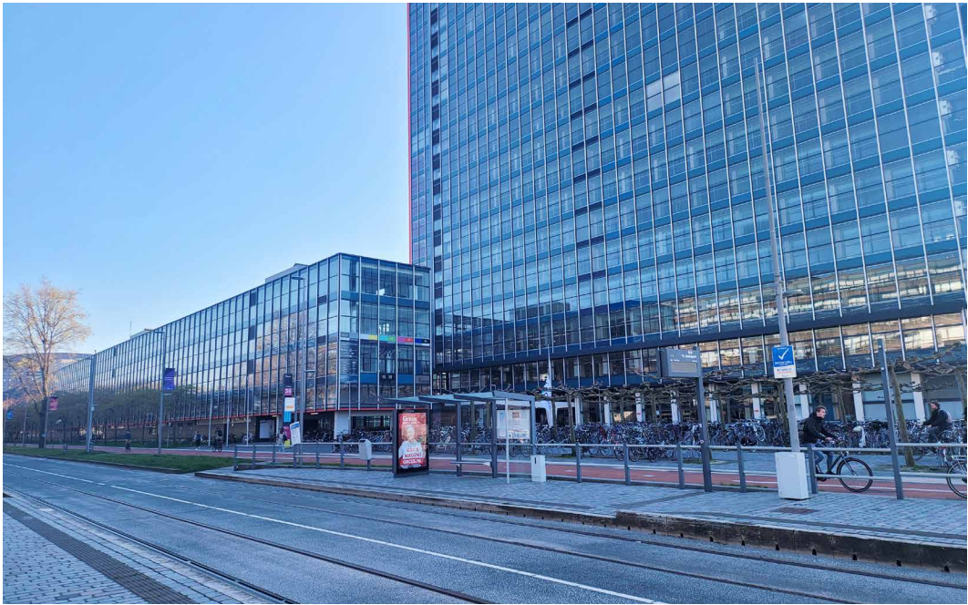
FIG. 3.1 TU Delft EWI Faculty Building (lowrise and highrise). (Photo: Azcárate-Aguerre, 2023)
