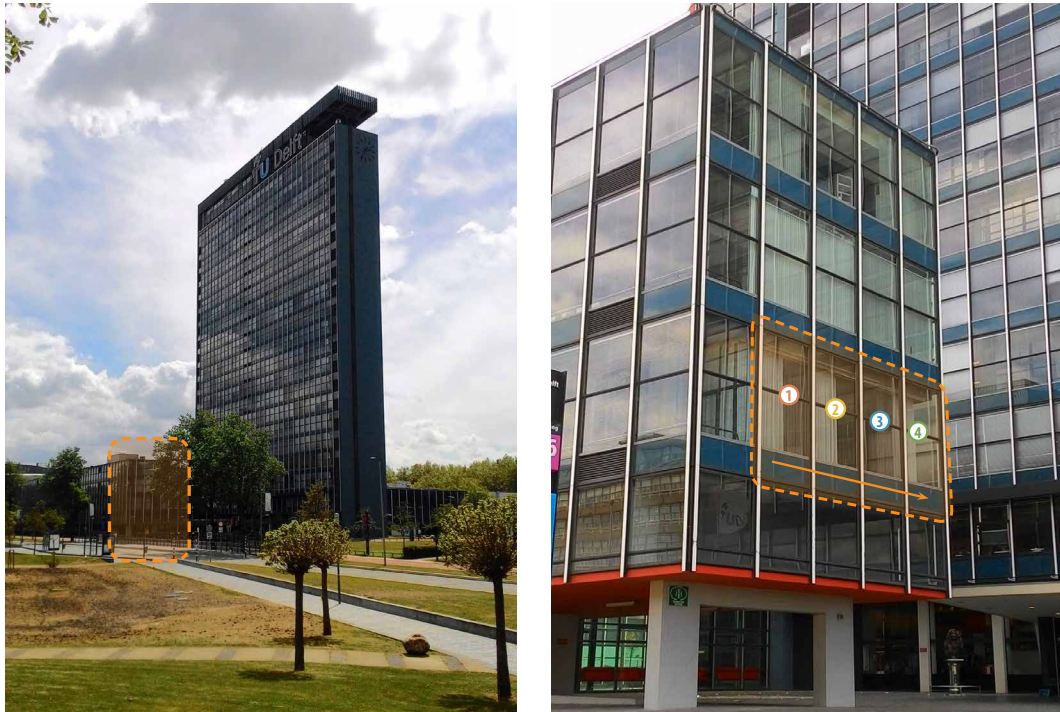
FIG. 3.3 Building complex of the EWI Faculty, TU Delft (left). Diagram showing location of the IFPSS pilot project on the north face of the complex's low-rise (right). (Photos: Azcárate-Aguerre, 2016)
