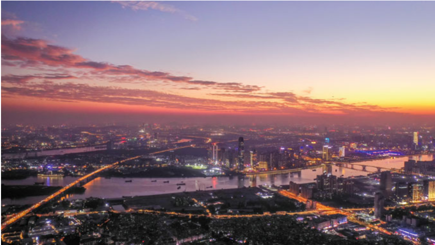
Fig. 5.1 In some parts of the PRD, there is barely any room left for the water. Photo Guangyuan Xie
