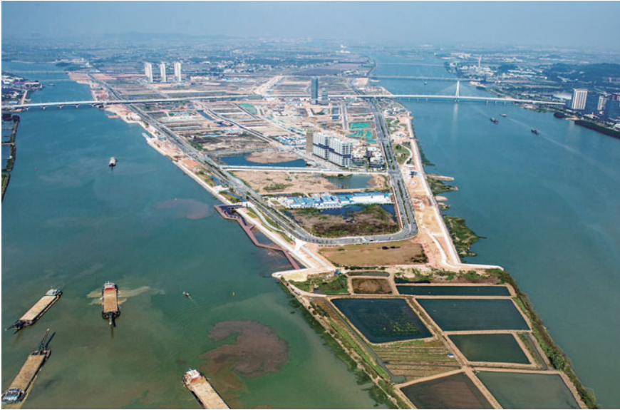
Fig. 5.24 Urban development of Nansha District. Photo Yimin Sun
