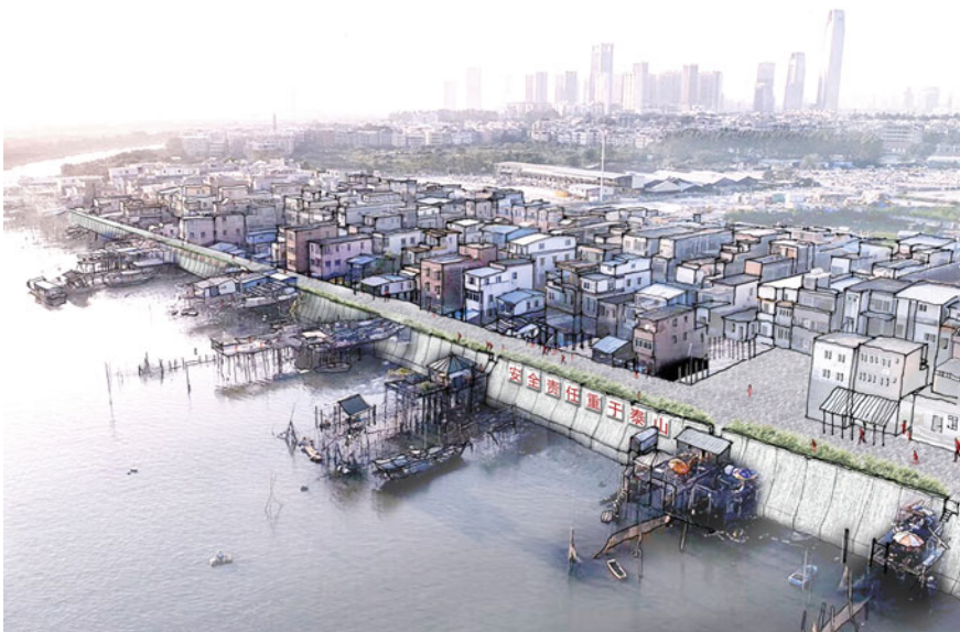
Fig. 7.8 Eastern portion of Pazhou Island. An existing fishing village is shown in the foreground, historic Pazhou village in the middle and newly constructed high-rise development on West Pazhou Island in the background. A new seawall is graphically superimposed and designed to protect the southern shore of Pazhou Island, which is currently unprotected during storm events. The jetties in the foreground have a partly religious as well as functional role (Drone picture by Aaron Xie; drawing by Bosselmann and Li 2019)
