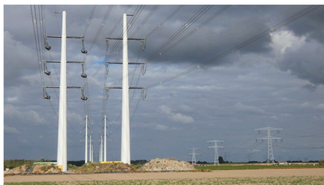
Fig. 4. Wintrack and Lattice pylons. Source: Hoogspanningsforum. https://www.hoogspanningsforum.com/viewtopic.php?f=12&t=1936 . Accessed 5–02–2023.
