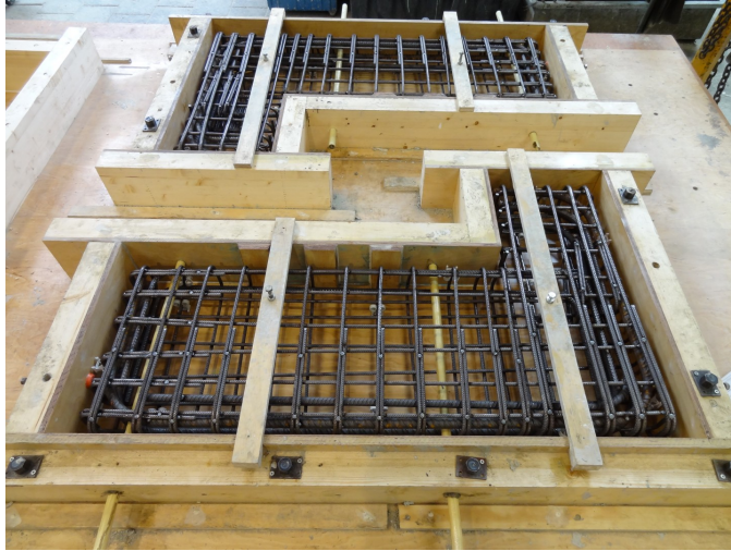
Figure 4.6: Construction of L-elements in the concrete factory
