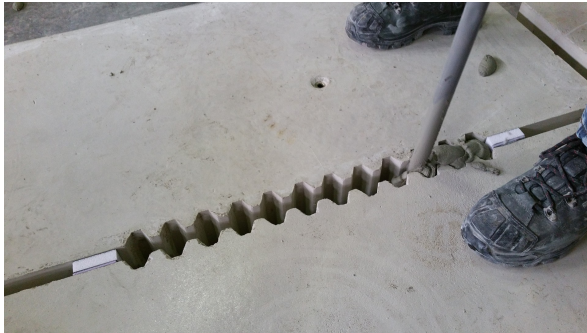
Figure 4.10: Inserting the mortar with a hose
