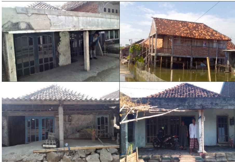
Fig. 4. Adaptation strategies through floor elevation (top-left), total house elevation (top-right), stone dike (bottom-left) and sand dike (bottom-right).
