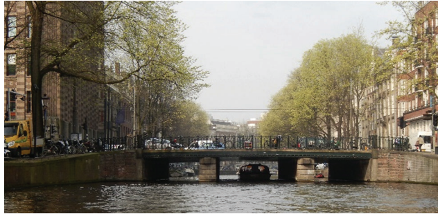
Fig. 1. Bridge on wooden pile foundation in Amsterdam/Netherlands
