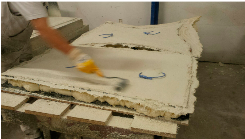
Figure 23. The finished sprayed GFRP being compressed with rollers to mitigate voids and air-bubbles in the GFRP.
