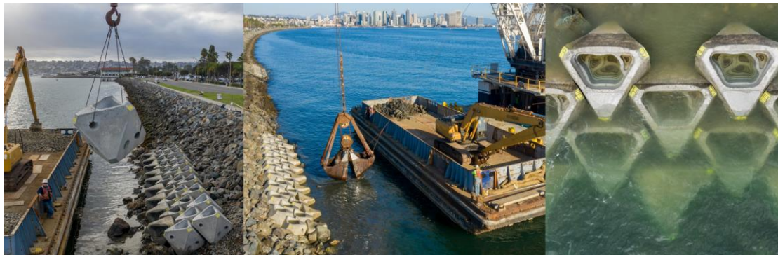
Figure 13. Installation of the Coastalock armour at PoSD, California, USA
