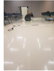
(c) Aligning floor markers
