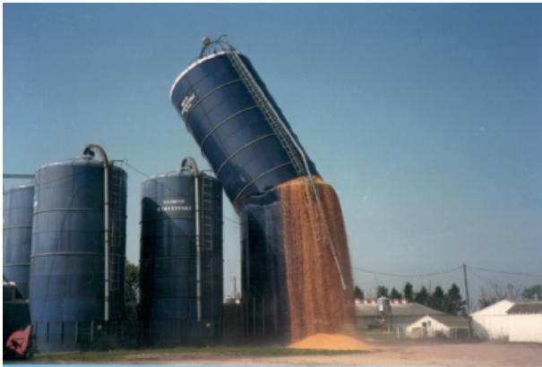
Figure 1.2: Grain silo in process of collapsing (Copyright Jenike & Johanson, Inc.).
