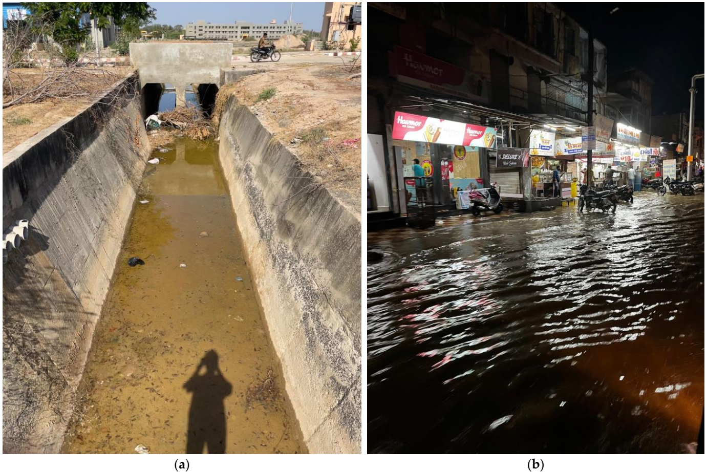
Figure 9. (a) The new 2 m drain to compensate for constructing the university campus in a droughty wetland (authors 2022). (b) Urban flooding after heavy rain in July 2022 (authors 2023).
