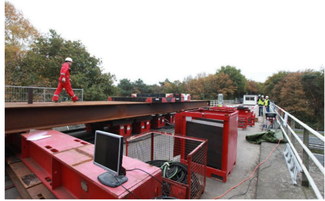
Figure 3. Proof load test on viaduct De beek, showing counterweights, steel distribution structure, and hydraulic jacks.
