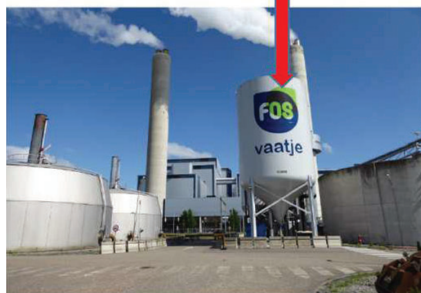
Figure 2: Magnesium recovery from a drinking water production reverse osmosis plant for struvite recovery from wastewater.
