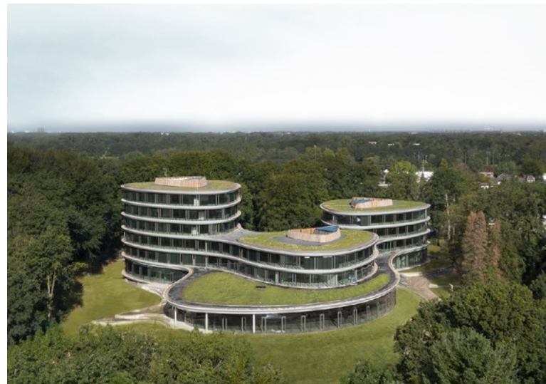
Circular construction with a focus on integration into the landscape (Triodos Bank, RAU architecten).
