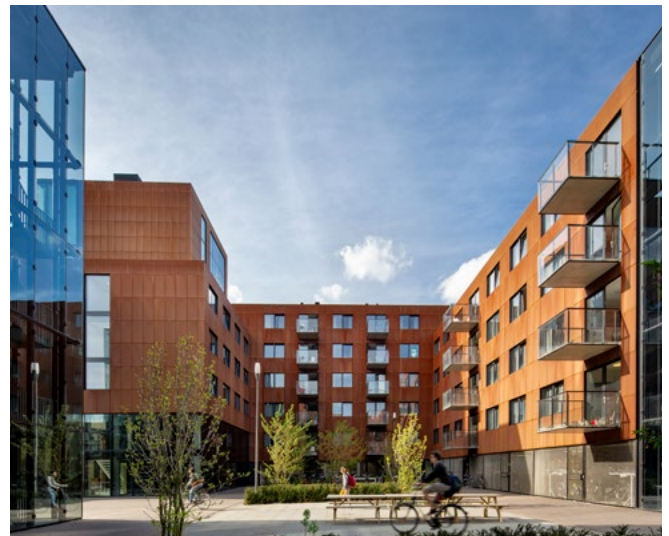
Shared residences on the campus, Schermerhornstraat (Cepezed).
