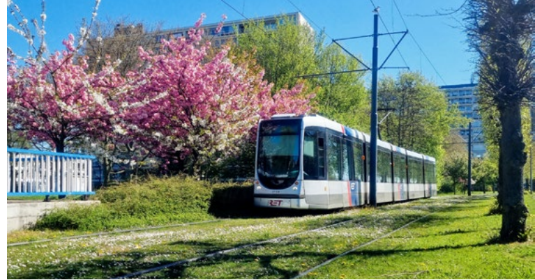
A green tram track in the Mekelpark takes care of integration into the landscape as well as capturing rainwater (Rotterdam).
