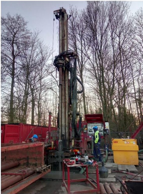
Drilling of DAPGEO-02 (500m)
