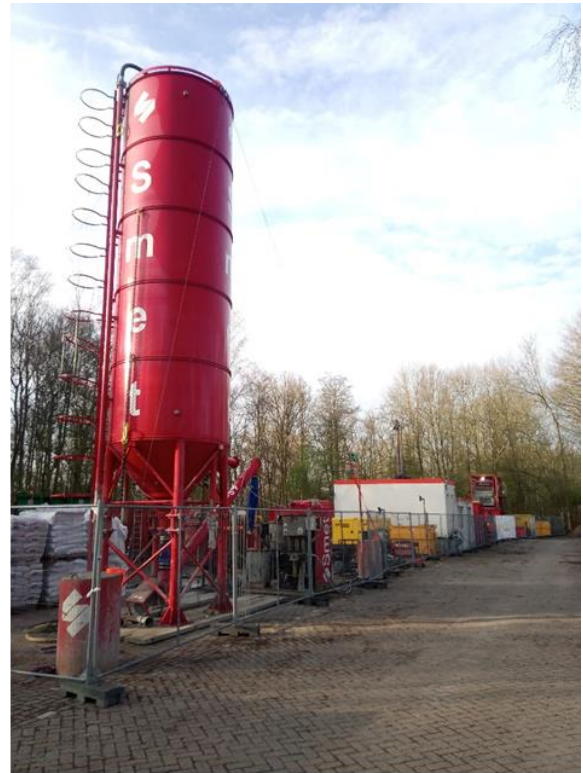
Drilling location DAPGEO-02 (500m)
