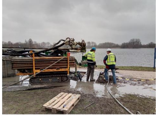
Drilling of DAPGEO-02-01B (50m)
