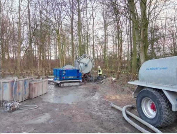
Grouting of DAPGEO-02 (200m)
