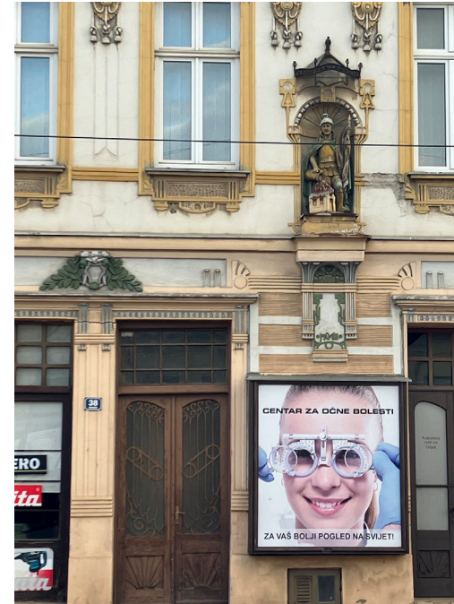
Fig. 3. Contemporary realities juxtaposed with past façade elements on Županijska ul (County Street), Osijek. Photo: Angeliki Sioli, August 2022.
