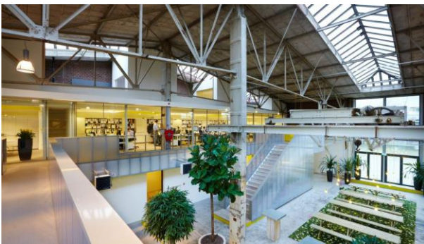
Figure 2: Reuse of existing factor for a modern office building (source: Imd/ Vincent Basler)
