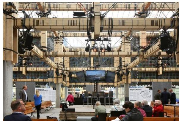
Figure 6: Temporary, demountable pavilion for the World Design Event during Dutch Design Week 2017 (source: Filip du Jardin)
