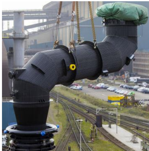
Figure 6-1. Scheme of current reflux chamber installation
