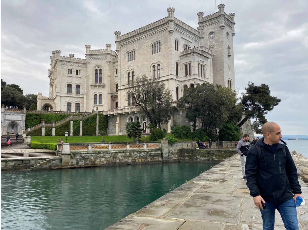
Villa Miramare (Source: Carola Hein)
