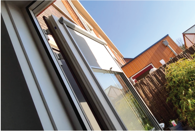
Figure 6. The retrofitted manual sunshade that can be drawn down to alter the light sensor readings.
