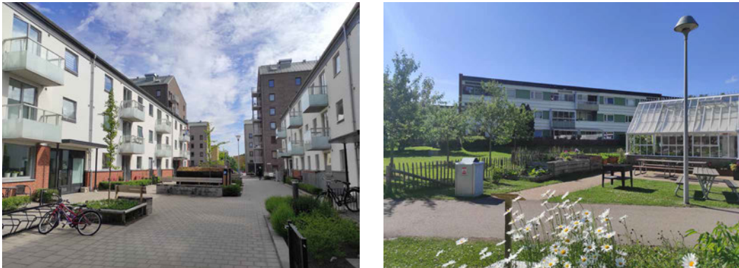
FIG. 5.6 Renovated and new buildings (left) and a new gardening house (right) in DrottningH
