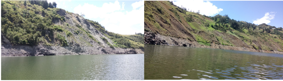
Figure 4.2: Examples of slopes around the Mazar lake, with visible alterations on the toe of the slope and signs of creep deformation.
