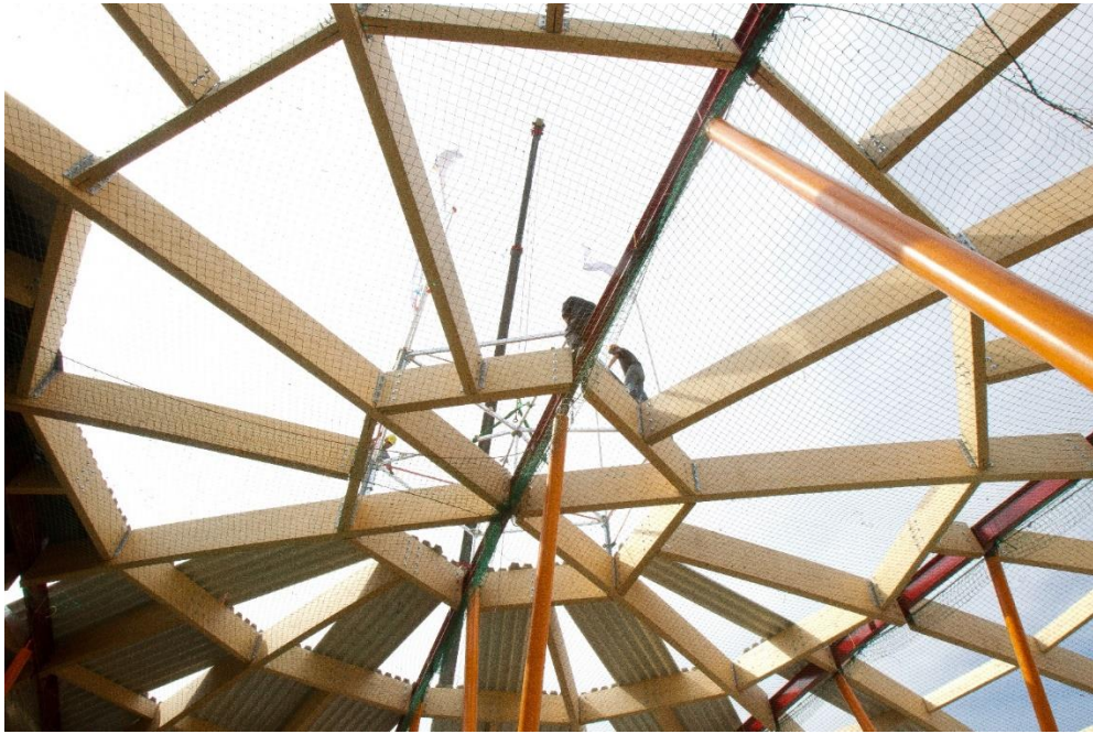
Figure 7: Timber roof under construction (Green Planet)
