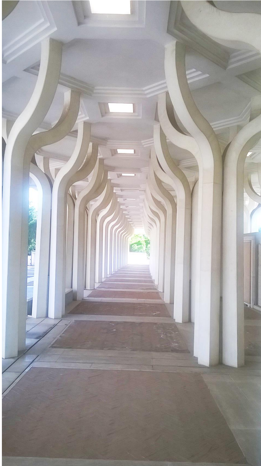
Figure 1: Arcade of a mosque with traditional Arab shapes using precast concrete (Rome)
