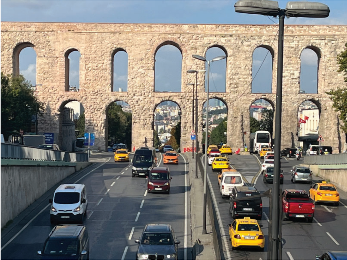
Fig. 1, The Valens Aqueduct (Bozdogan Kemer) in Istanbul, Source: Mariëtte Verhoeven, 2022, CC BY-NC-ND 4.0
