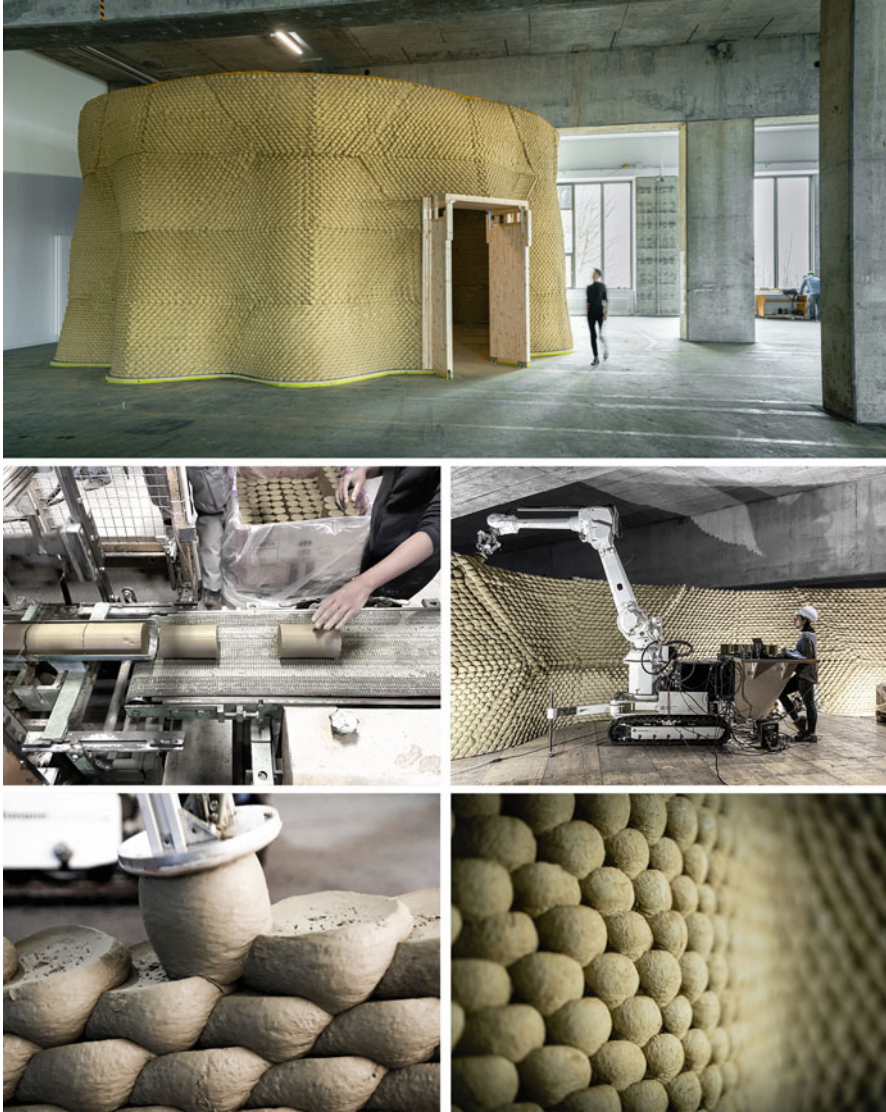
Fig. 9.3 (i) The Clay Rotunda is a cylindrical structure constituting the outer, soundproof shell of the electroacoustic auditorium SE MusicLab. (ii) The soft bricks were produced externally with an industry partner. (iii) The robotic pressing process was realised with the IF, which could be relocated on a temporary scaffold to realise a two-story structure. (iv) Detail of structure showing the bonding and interlocking between adjacent elements. (© Gramazio Kohler Research)
