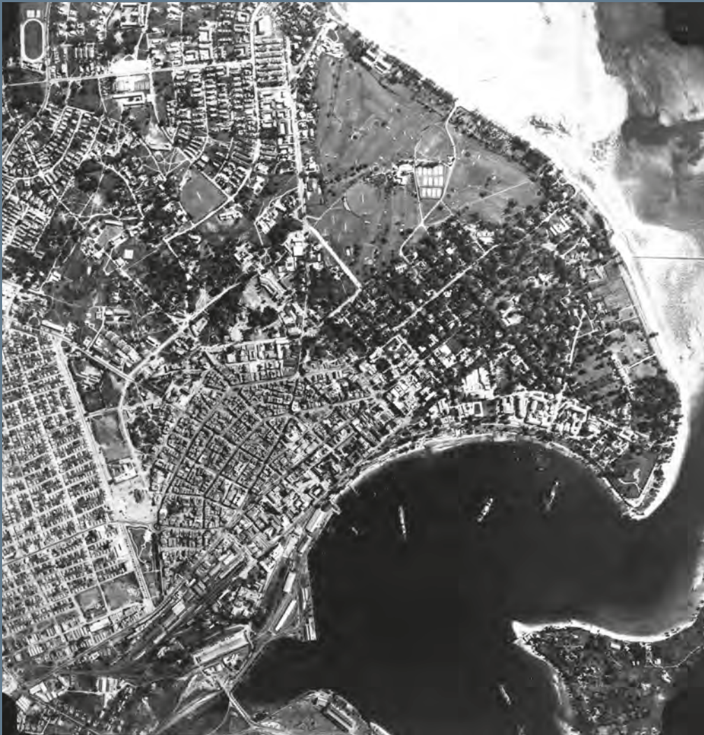
Air view of the central area Dar es Salaam Tanzania, 1967
