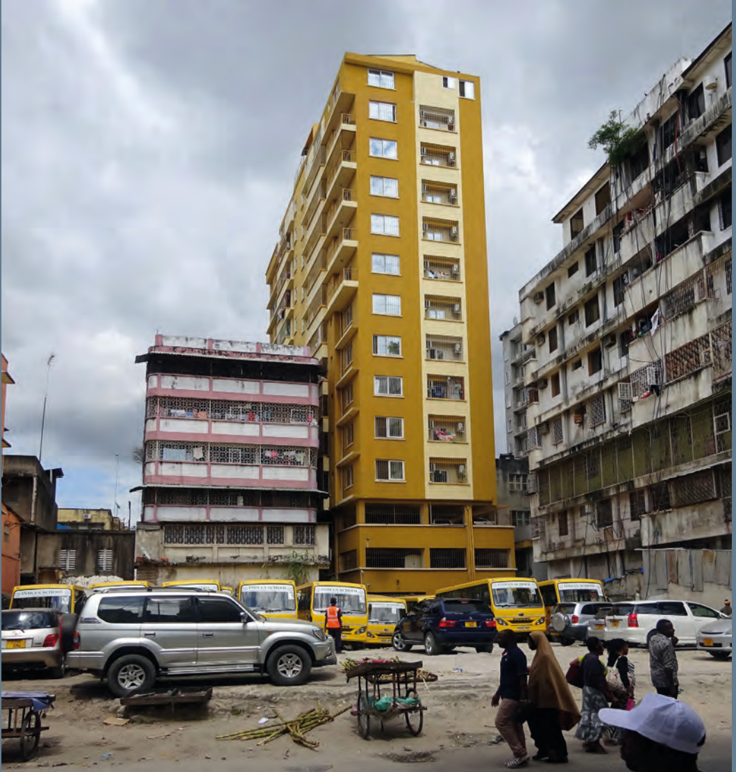
Central Dar es Salaam under redevelopment
