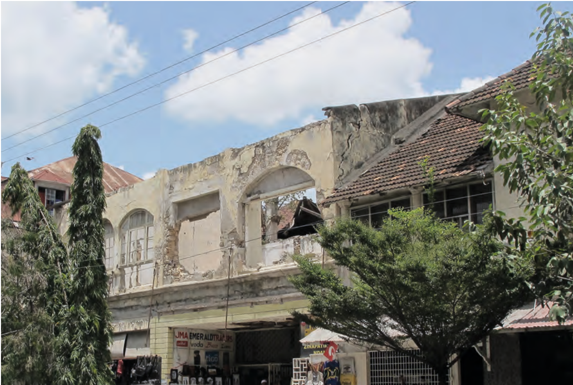
Demolition of old buildings in Dar es Salaam
