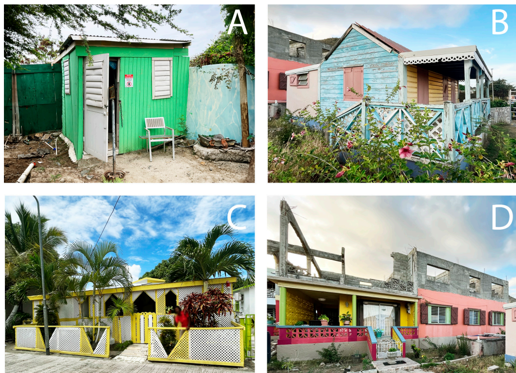
Figure 3. Impressions of different types of self-organized housing on St. Martin. (A) small housing unit at Pond Island using temporary materials; (B) light balloon-frame timber house with a porch and concrete extension in the back; (C) pre-fabricated concrete house with porch built as an extension; (D) house built with concrete blocks with an unfinished upper floor. Source: authors.
