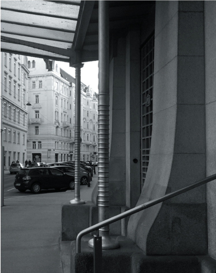
5.04 Aluminium clad columns to resemble screws at the entry canopy. Photograph by Eireen Schreurs.
