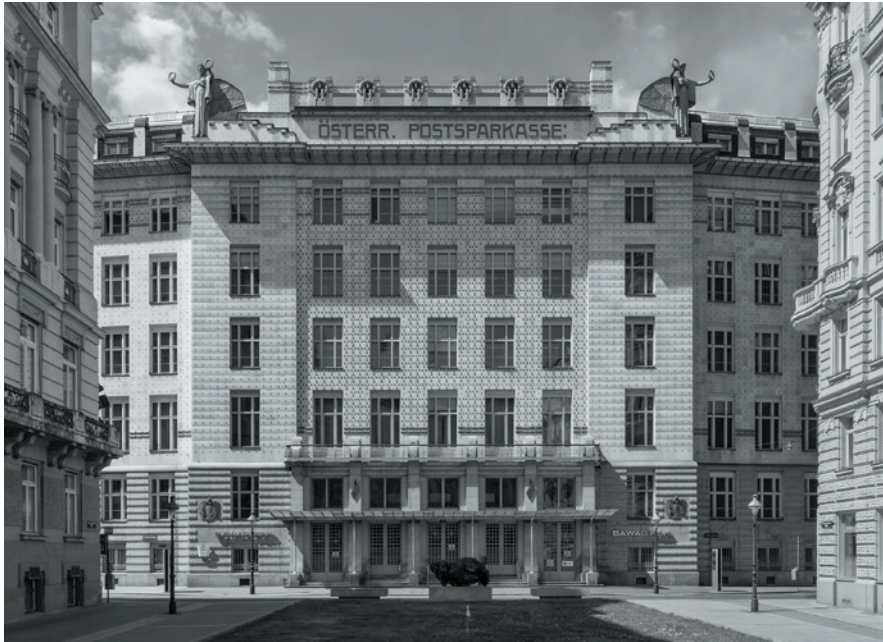
5.01 Front façade of the Postal Savings Bank, with a pattern of bolts. Photograph by Thomas Ledl, CC BYSA.
