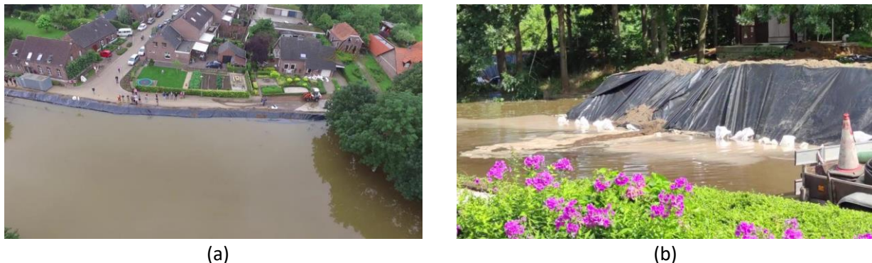
Figure 5: (a) Emergency dike near Horn with the location of the subsequent breach to the right (YouTube, 2021a), (b) the start of the breach (YouTube, 2021b).
