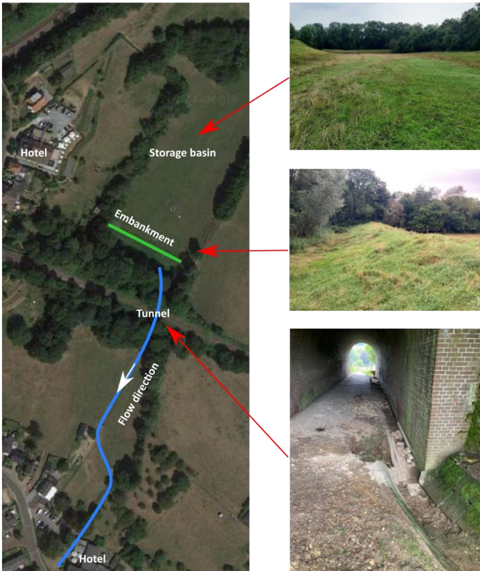
Figure 13: Location of Ransdaal storage basin near Schin op Geul (left) and images of the basin, the dike/embankment, and the erosion in the tunnel downstream (photographs provided by Bas Jonkman, TU Delft).
