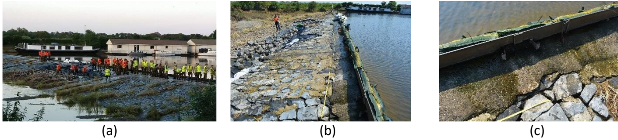
Figure 10: Barrage near Bosscherveld: (a) emergency repairs with the assistance of the army (photograph Wilbur van Beijnen, Directorate-General for Public Works and Water Management), (b) overview of defence after repair (high-water marks still visible from the vegetation in the background), (c) detail of anchoring of steel edge.
