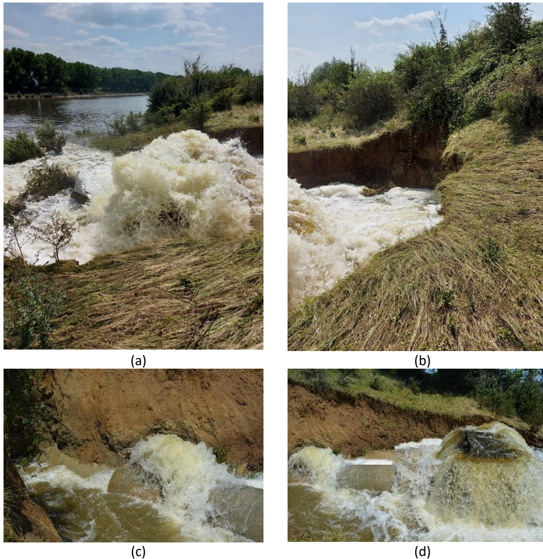
Figure 11: Zeven Ellen Waterlaat near Horn: (a, b) situation on 21 July (photographs Erik Bijlsma, Directorate-General for Public Works and Water Management), (c, d): situation on 23 July with a level of approximately 1.95 m below the peak water level in the retention area.
