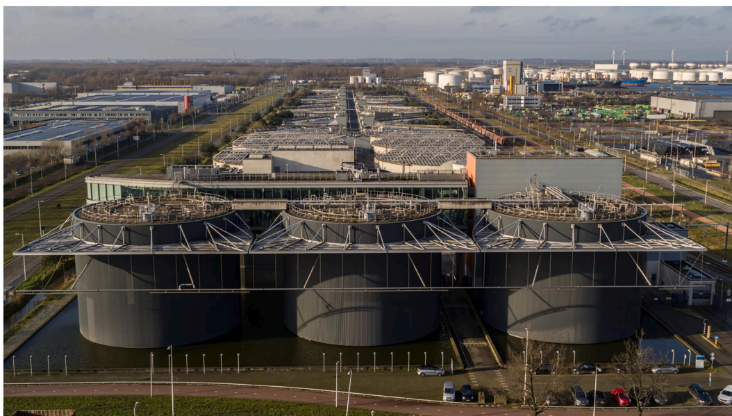
Fig. 4. Amsterdam West WWTP (Source: Waternet).
