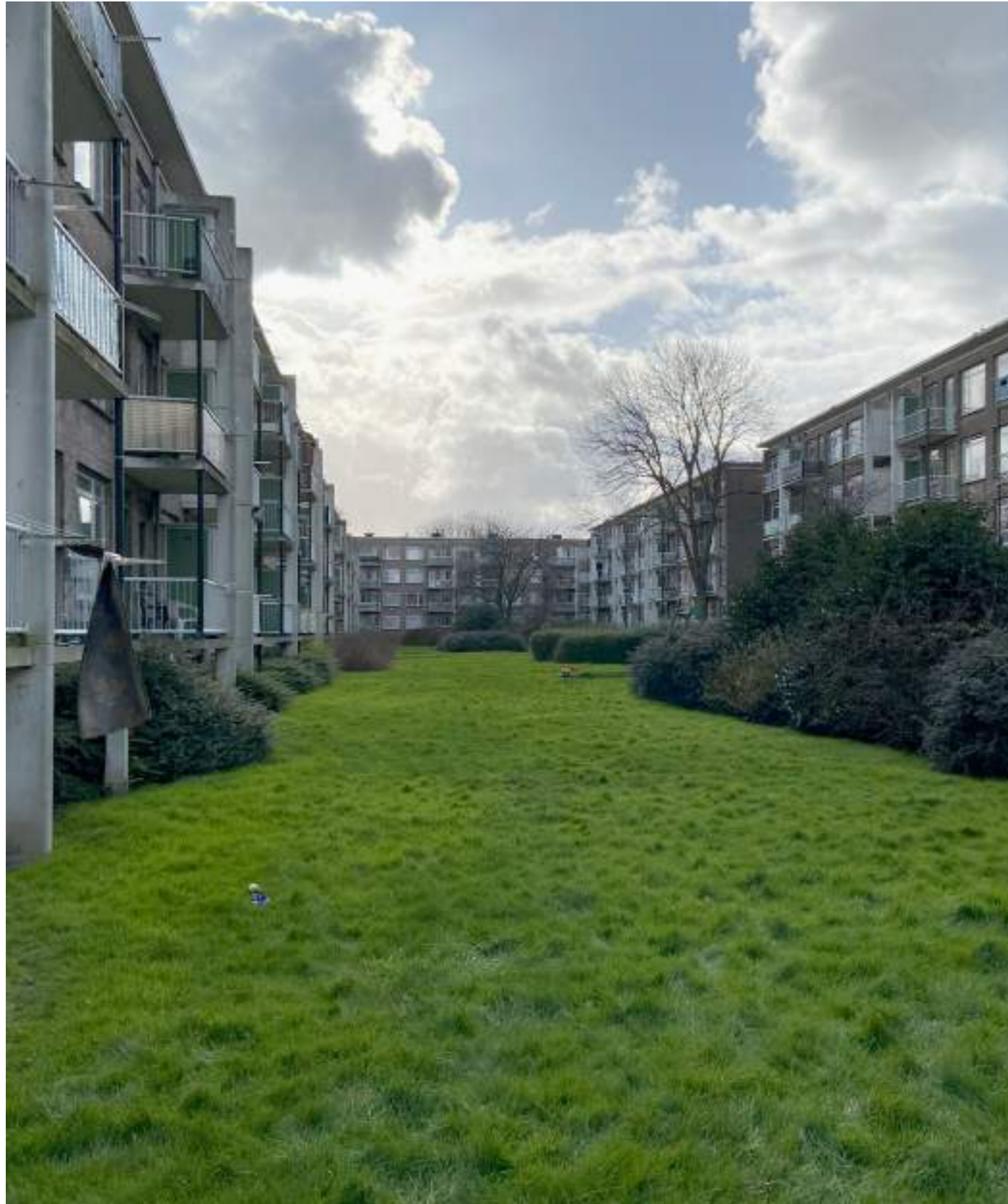
Figure 17. A typical courtyard from Dudok's urban design – an elongated courtyard tightly enclosed by a group of residential building blocks, distinguishing the communal realm and urban realm.
