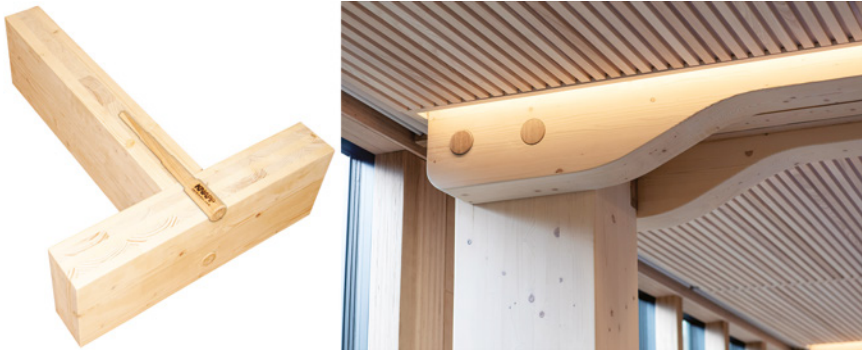
FIGURE 12 Pre-dried dowels. (Left) Mateo Timber peg (Knapp GmbH). (Right) Custom beech dowels utilized in the Bjergsted Finace Park (Sindre Ellingsen)
