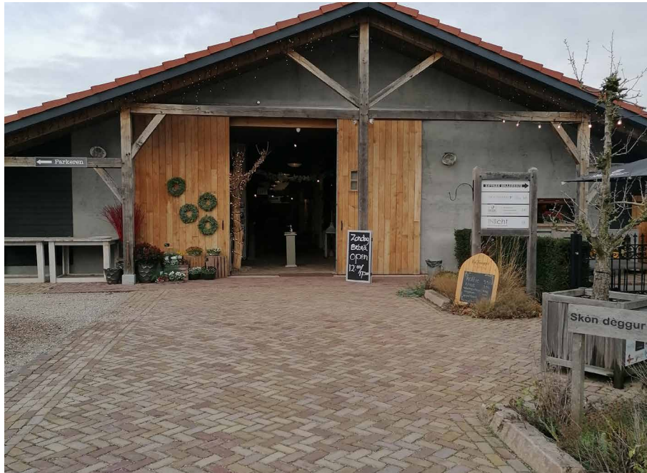
FIG. 4.3 The re-used farm building of Mouthoeve . Source: First author (2020).
