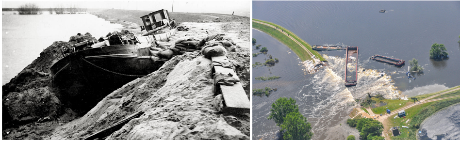
Figure 1.1: (left) Successful breach closure with vessel Nieuwerkerk aan de IJssel, Netherlands 1953 and (right) unsuccessful breach closure with vessels Fischbeck, at the Elbe river, 2013 (Mauritius Images / Alamy Stock Photo)
