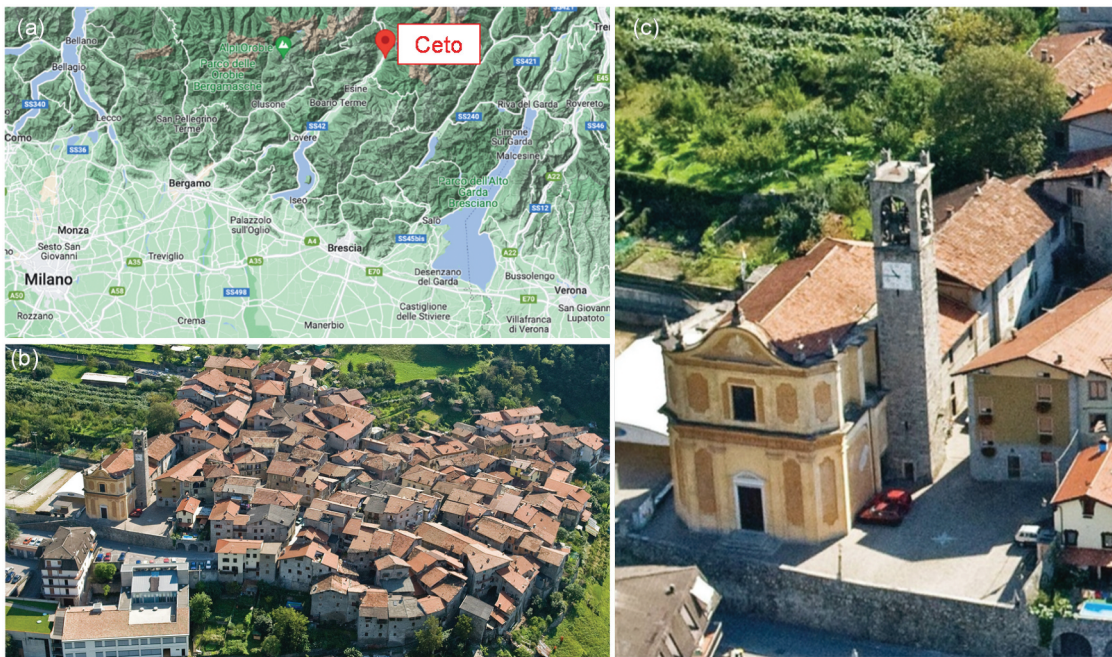
Figure 1. (a) Location of the analysed church in the province of Brescia; (b) position of the church in the town of Ceto; (c) case-study building.
