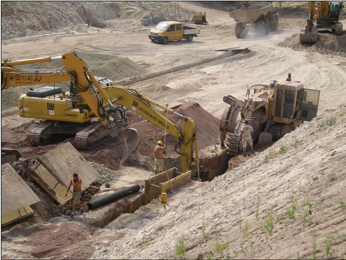
Figure 1-1: Earthwork in Germany (source Wikimedia).
