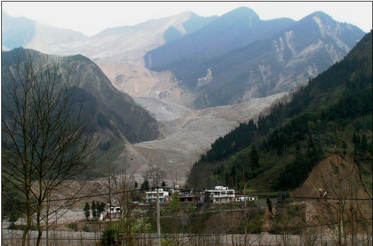
Figure 1-5: The Wenjiagou landslide (blogs.agu.org).
