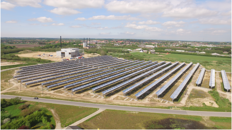
Figure 1.5: CSP ORC power system manufactured by Turboden. (23)
