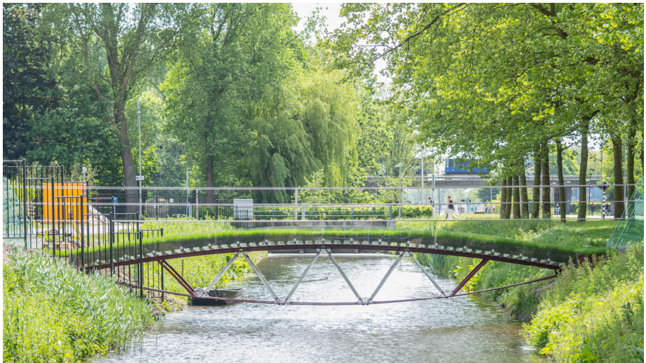
Figure 2: The Glass Truss Bridge. Note that the most left and most right diagonals are of steel. photo by Frank 'Graphdude' Auperle.
