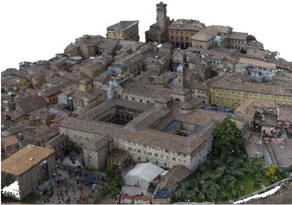
Figure 4. 3D point cloud obtained from the integrated survey.
