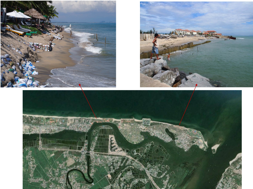
Figure 1.1: Erosion problem at Cua Dai beach
