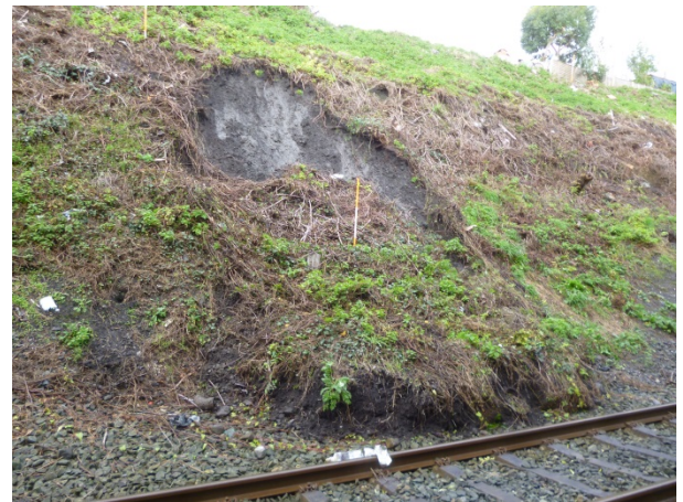
Figure 4. Examples of typical landslides on Irish rail network: a) on embankment, b) and c) on cutting
