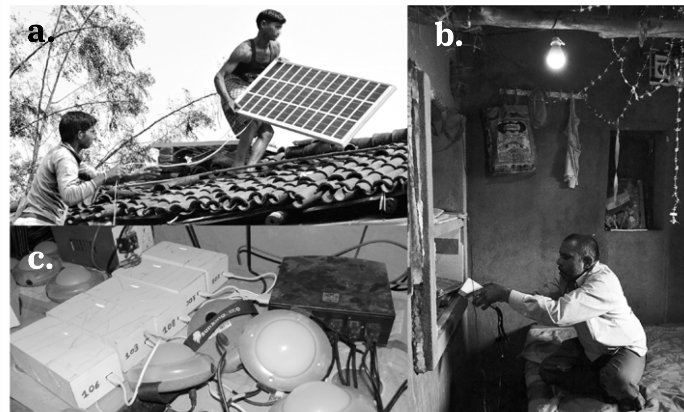
Figure 5 a, b, c, d. Photo: Abhigyan Singh. Energy Distribution Infrastructure. (a) Solar Panel. (b) Energy Router, Power banks, and Solar Lanterns. (c) LED Bulb and Power bank. Each solar item was imprinted with a unique numeric code to facilitate tracking of energy exchanges.
