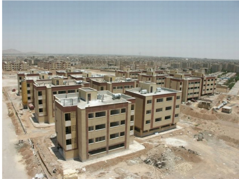
Figure. 5.4. Residential development south-west of Tehran's boundaries
