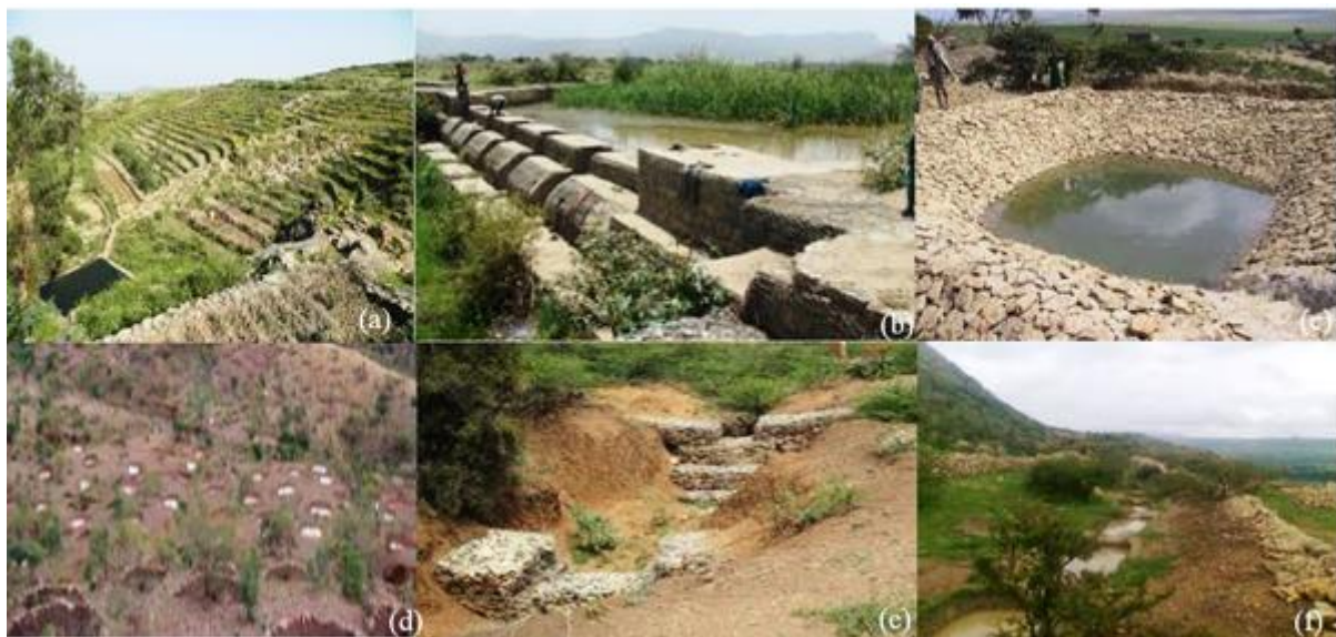
Figure 7.2: Physical SWC interventions in the Geba catchment of the Upper Tekeze headwaters: (a) terraces, (b) check dams, (c) water harvesting structures, (d) percolation ponds at the top of hills, (e) gully rehabilitation using gabion, (e) deep trenches at the bottom of hills (sources: (Woldearegay K & Tamene L, 2017; Yosef & Asmamaw, 2015).
