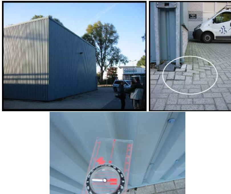
Fig. 4.21. A possible double-bounce reflection (PS velocity -9 mm/year). Since the pavement around the building is subsiding, the SAR reflection is likely to be a curb-to-wall reflection. The orientation of the building towards the satellite look direction confirms that a double-bounce reflection is possible.
