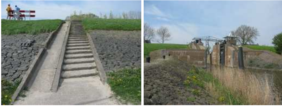
Fig. 4.23. More PS targets in the Netherlands: (left) dike covered with basalt blocks that is a distributed PS, (right) sluice that is most likely represented by a multi-bounce reflection.
