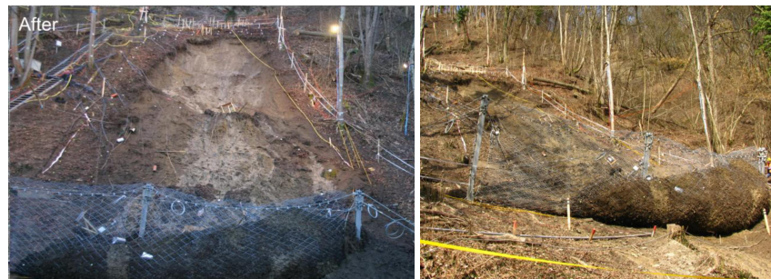
Fig. 13: Photographs of the Ruedlingen slope sediment after the debris flow of 17 March 2009. Note the deformation of the debris that accumulated in front of the barrier. Reproduced from [3].
